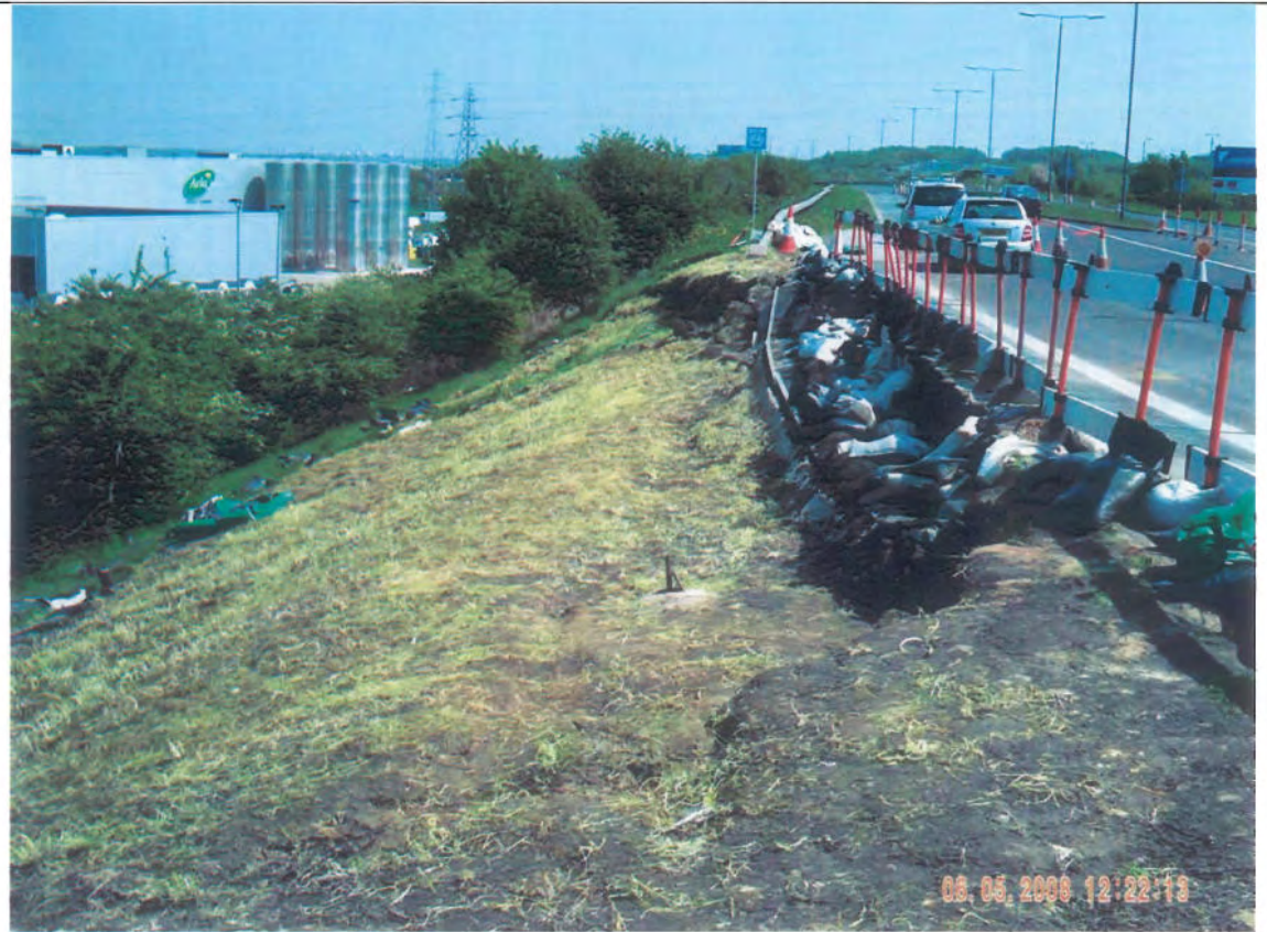
▲ Photograph 3 – The cracked footway looking west (May 2008).
